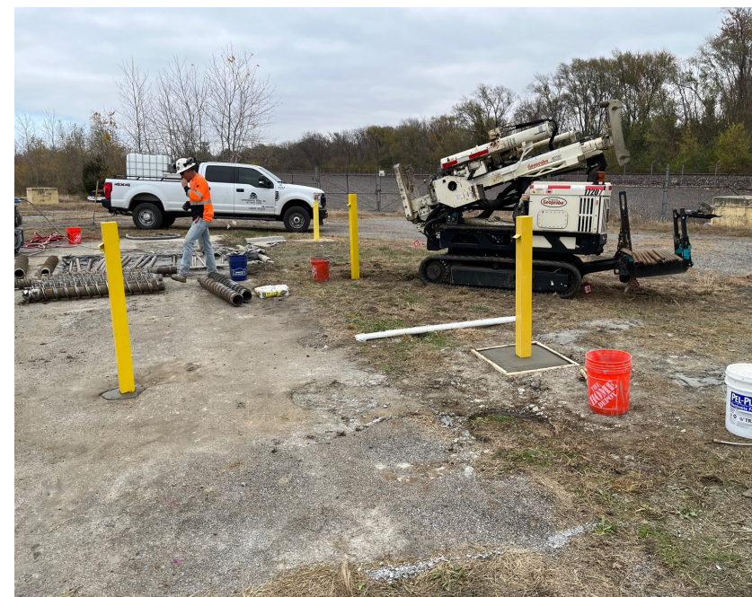
Drilling and installing monitoring wells at the Facility
