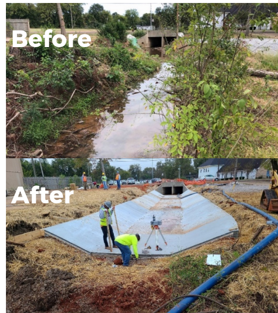
Stormwater drainage ditch looking southeast towards Waterworks Road
